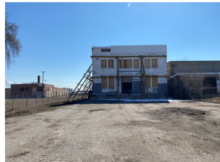
7 View of the existing Salt Lake Mattress Building looking south from 300 South.
