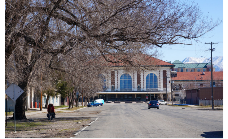
4 View of the Rio Grande Depot looking east from 300 South.
