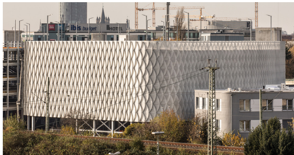
Figure 4.18: The Parking Garage Facade P22a designed by Wulf Architekten in Koln Germany successfully creates a facade that is light, transparent, and playful, both during the day and night.
