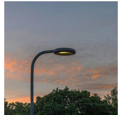
Figure 3.27: Exterior street lights that adhere to dark sky standards help mitigate light pollution and disruption of circadian rhythms.
