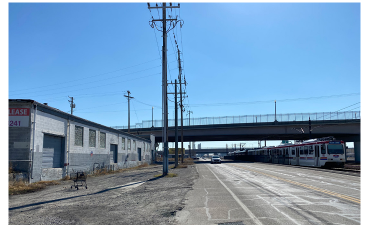
6 View of WRR Industries building to the east, TRAX on 600 West to the west, and the 400 South viaduct in the background.
