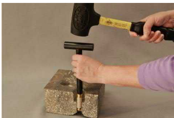
Figure 3. Flush-mount installation.
