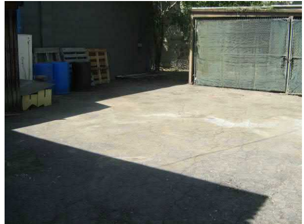
Photo #14 Drum storage (empty); however, note the drum imprints from long term storage and staining in the area.
