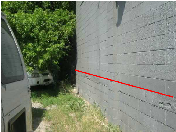
Photo #15 Red line shows approximate area where spent etchant was seeping from the plating room to the exterior of the building.
