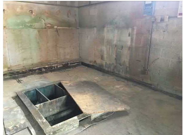
Photo #4 View of the sump, in the area of the former waste water treatment area.
