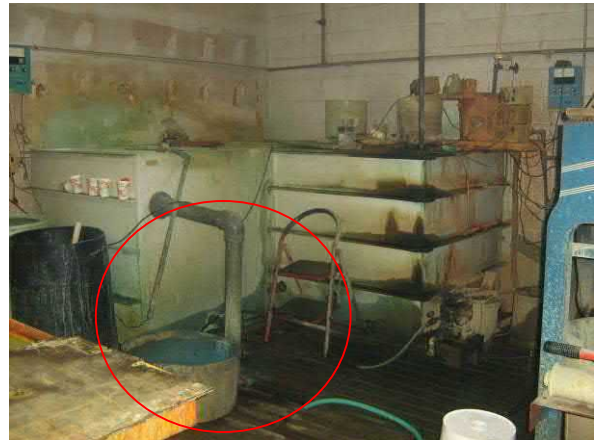
Photo #12 Sump location is underneath the wooden panel flooring. Pipe is showing the connection between sump and WWTS.
