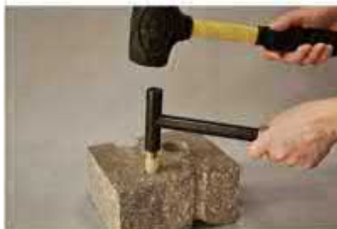
Figure 5: Installing the Vapor Pin™
