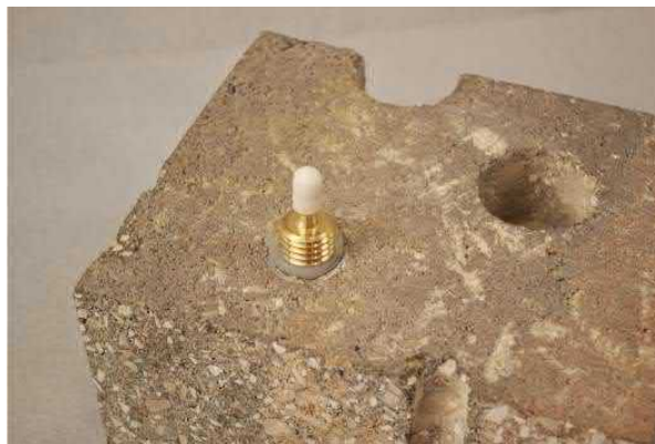
Figure 4. Installed Vapor Pin™.
