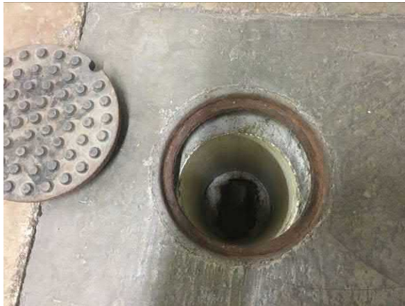
Photo #3 View of the access to test the wastewater going to the municipal system in the general room.
