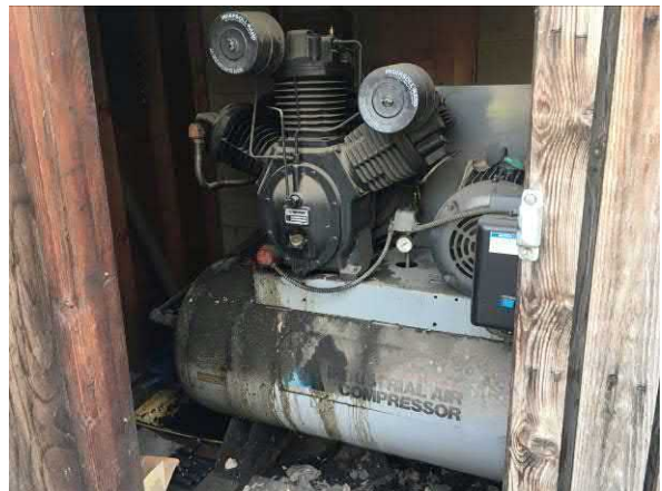
Photo #10 Air compressor, staining observed.
