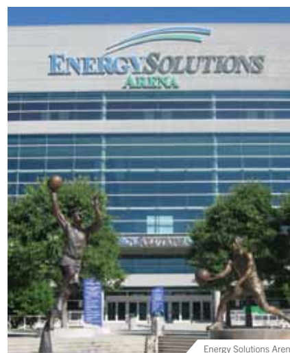
Energy Solutions Arena
